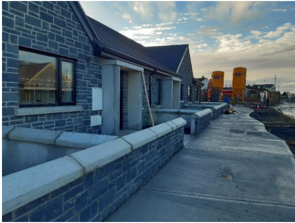
Level access in Fana Bhui in Tuam
