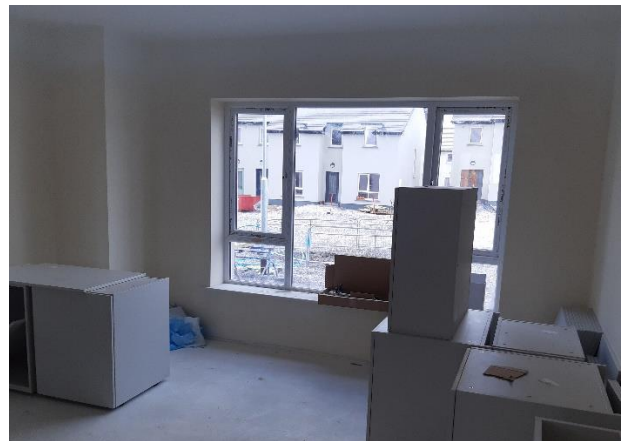
Larger windows = high light levels, Tubber Rd, Gort
