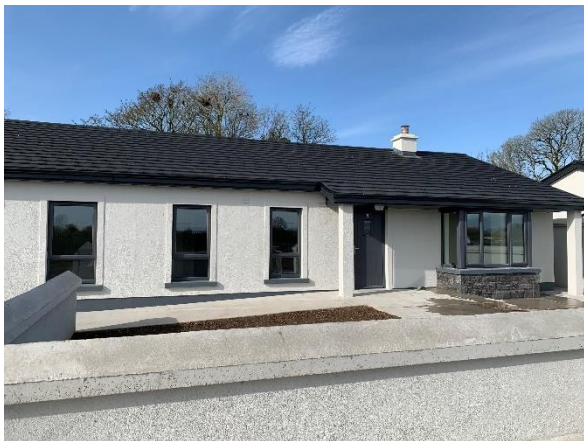
Level Access Footpaths in Craughwell
